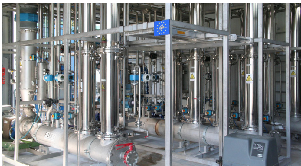
The 'PVClean' ultrafiltration facility in the S-PVC plant Knapsack
